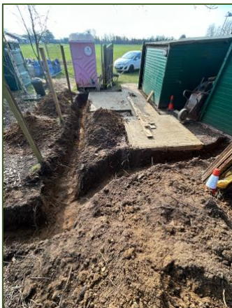
Sewer pipe trenches to toilets and Clubroom (for sink)
