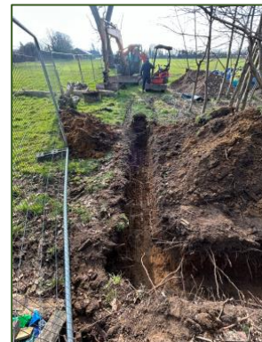
Sewer pipe trench to STP
