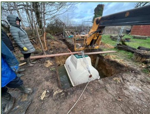
Sewage Treatment Plant being installed
